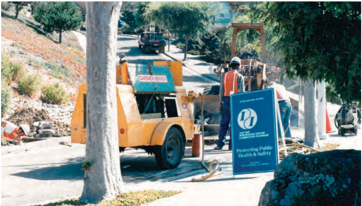
Infiltration and Inflow repairs on Douglas Drive in El Cerrito
