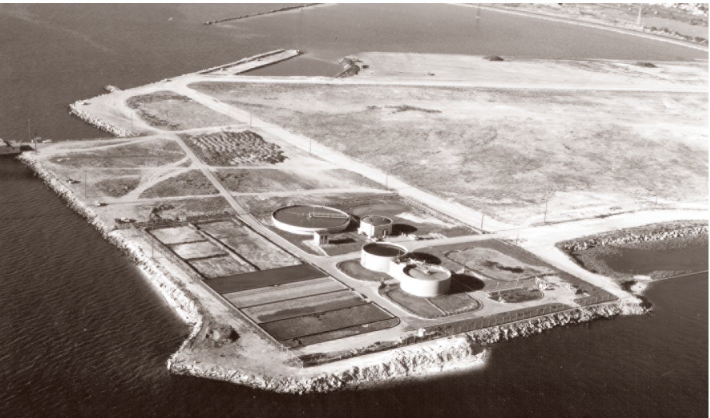
Point Isabel primary treatment plant
