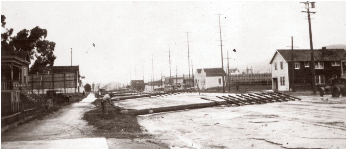
Telephone poles lie uprooted after a rain and wind storm in 1927. The view is on San Pablo near Fairmount Avenue looking towards Albany. El Cerrito Historical Society, photo courtesy Louis L. Stein.
