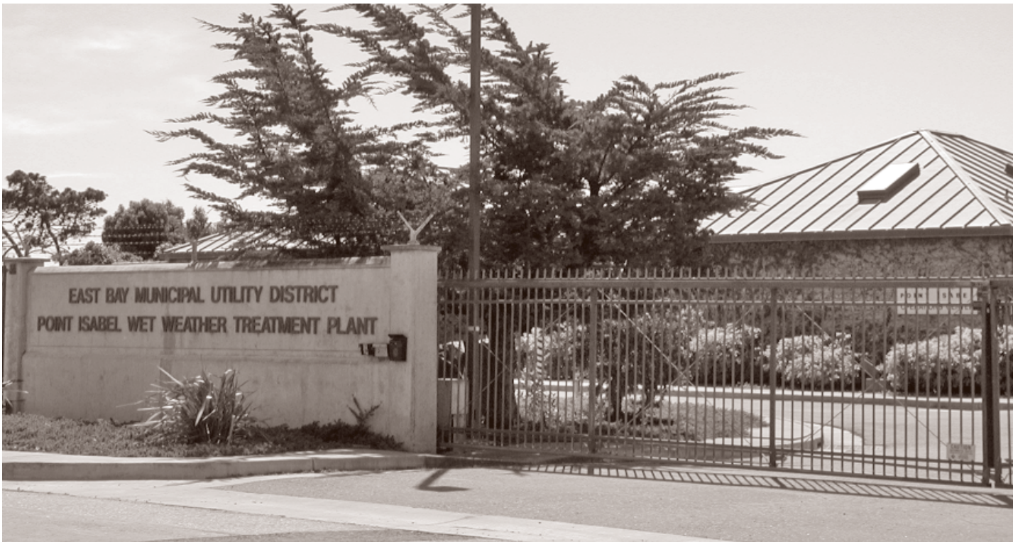
In 1977, Stege sold its Point Isabel station to EBMUD. Today the station operates as an EBMUD wet weather treatment plant. Photo by Rosalie Blazej
