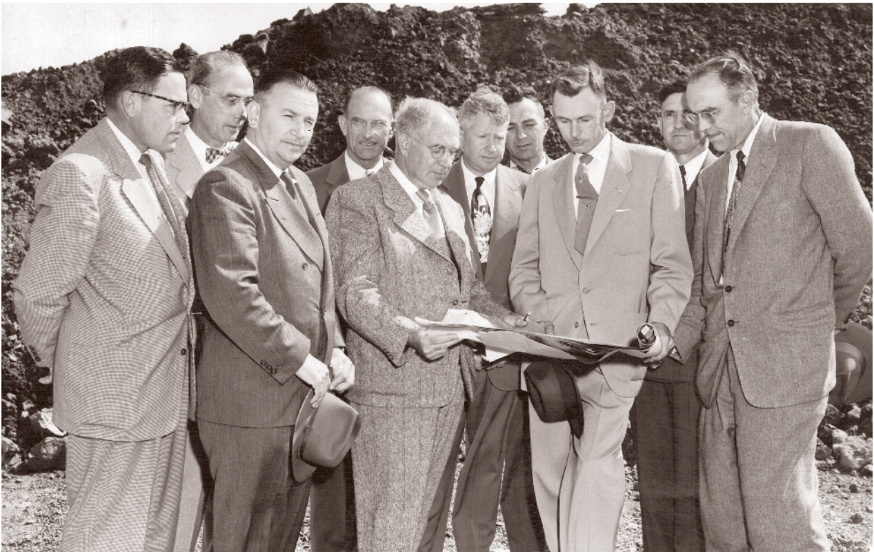
The plant’s ceremonial groundbreaking took place in September 1953. Present were Stege director Tubby Snodgrass, Tom McMorrow, Stege director Walter Weyand, Al Baxter, and El Cerrito city councilman Ed Valentino
