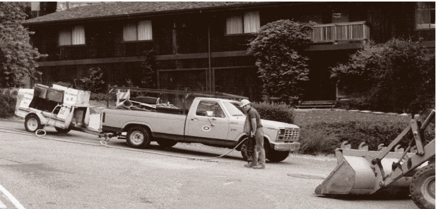
Infiltration and Inflow rehabilitation work
